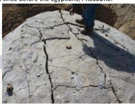
Sylentmite in the holes. When the bolder is cracked and Sylentmite has finished it's reaction, you're left with a non-toxic powder that can simply be washed away and is biodegradable.
