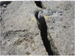
The holes were filled with Sylentmite and were all left overnight to break up these boulders, but dependant on ambient temperature and the strength of the Rock/Concrete you're breaking, cracks can appear after around 45 minutes. Notice how the break has appeared just through the expansion of Sylentmite!
