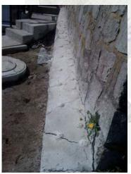
After preparing an easy Methodology statement, a drill pattern was designed, drilled, Sylentmite was mixed and packed into the holes and left to do its work overnight.
